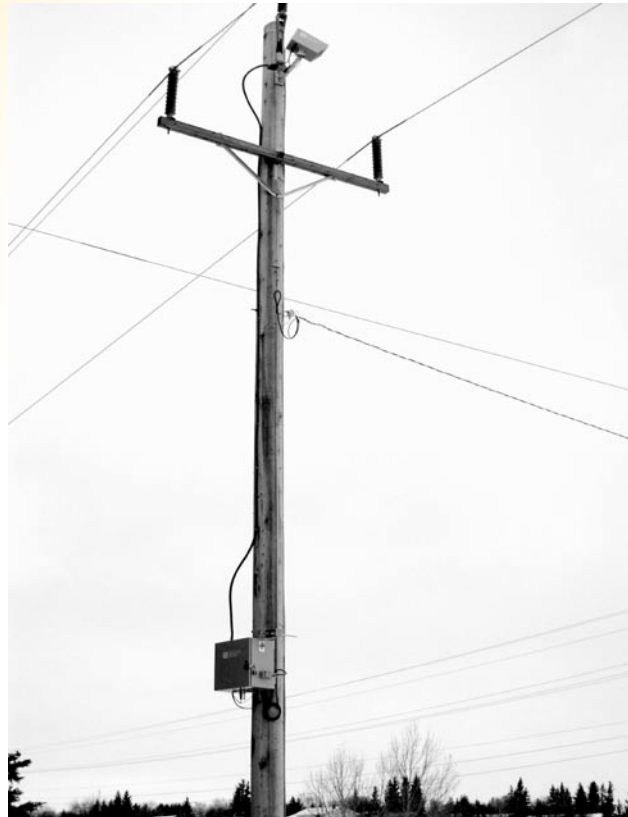
Figure 1 Ice system set-up on 66kv line
